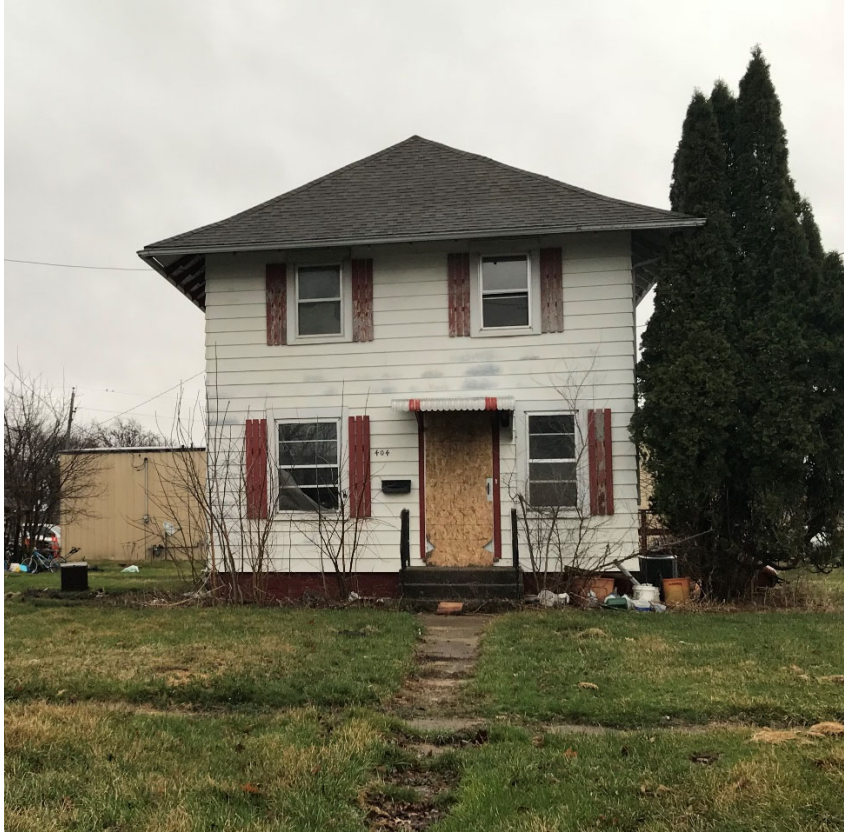
Figure 2 Example No. 2 - Boarded up door, potentially abandoned property.
